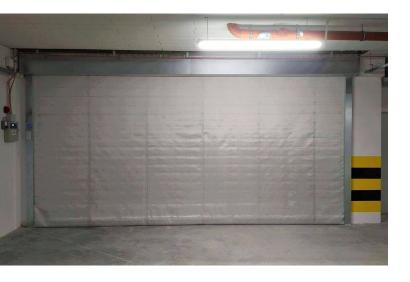
The El Fire curtain is a system for an absolute thermal insulation. It reduces the thermal radiation to minimum level and keeps the surface temperature below the 140 °C, for at least 60 minutes.
